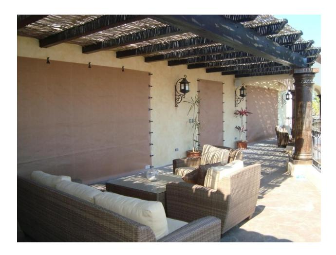
In the above application, all three openings have a side to side attachment span. However, you will note that only the two longer openings have supplemental anchors on the top. The order will provide for the required 9 Clips/Anchors on each of the sides (54 total) and the optional top Clips/Anchors (6) should be added to your order.
