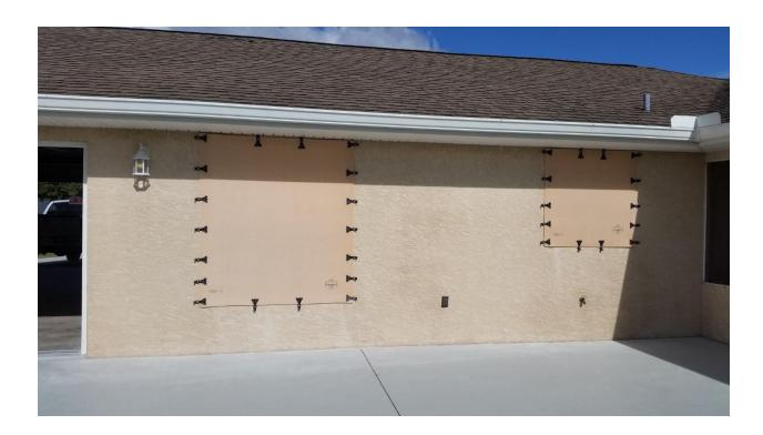
In the above application, both window attachment spans are side to side and the two additional anchors top and bottom, although not required, were desired by the homeowner. In this application, the order will provide for the required 24 Clips and anchors on the sides. The optional supplemental anchors (4 or 8) should be added to your order.
